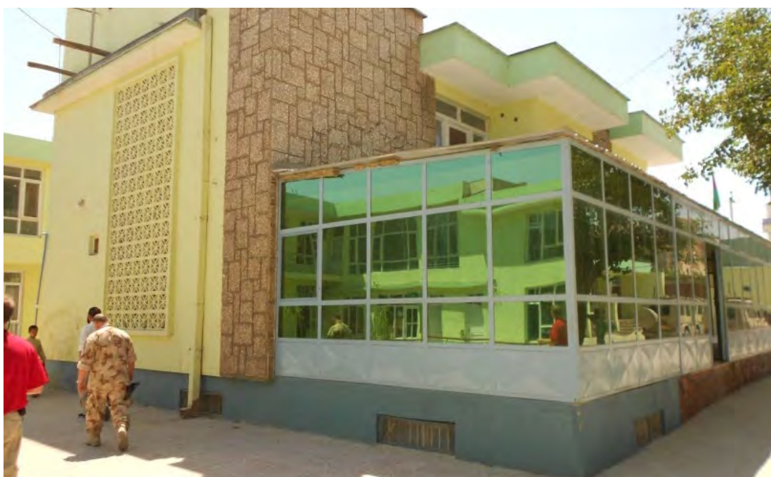
Figure 28. Provincial Headquarters AUP Clinic, Mazar-e-Sharif Source: DoD IG-SPO
